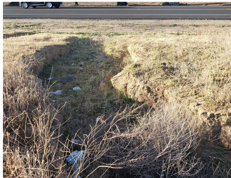
Photograph 4: View facing approximately southeast depicting the location where AF-2 connects to the roadside ditch segment of AF-1.
