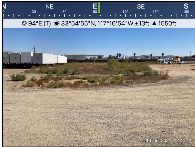
PHOTO 3: VP2 and VP1. View is southeast toward culvert (October 14, 2021).
