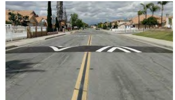
Speed humps are a common traffic calming measure in residential areas.
