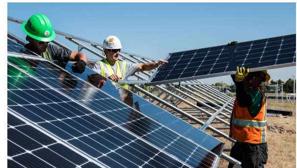
MVU and other regional and state partners offer rebates and assistance to help customers install energy efficient upgrades such as solar panels.
