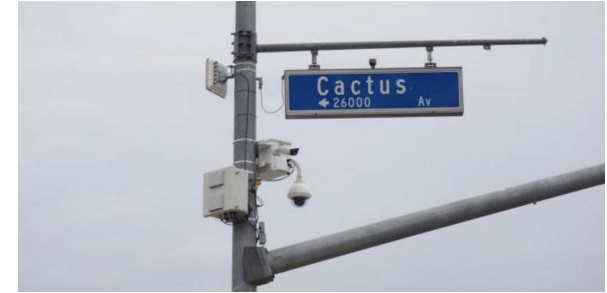
ITS allows the City to monitor different locations strategically and adjust traffic signals to improve flow.
