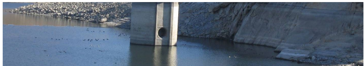
Seismic retrofit of the Perris Dam. Photo credit: California Department of Water Resources, 2019.
